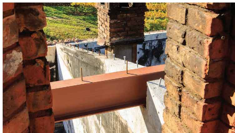
A view from the top of the Farmhouse. All iron beams supporting the Italian roof tiles were destroyed in the Glass Fire and were replaced.
